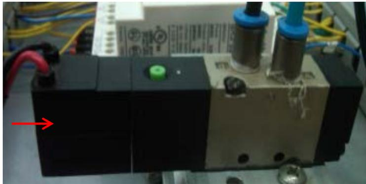
Gambar 7. *Selonoid valve 5/2 spring return*
